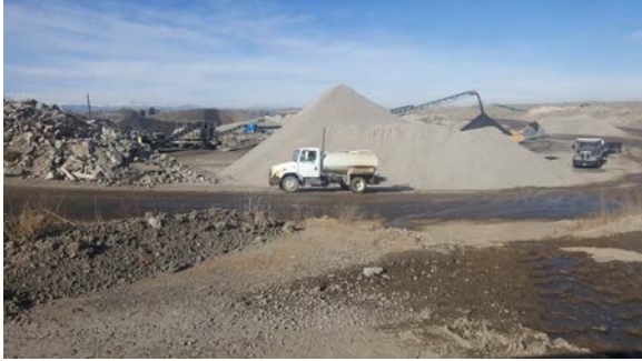
View of concrete crushing process (background) looking southwest. View of damp road conditions and water spraying truck (foreground).
