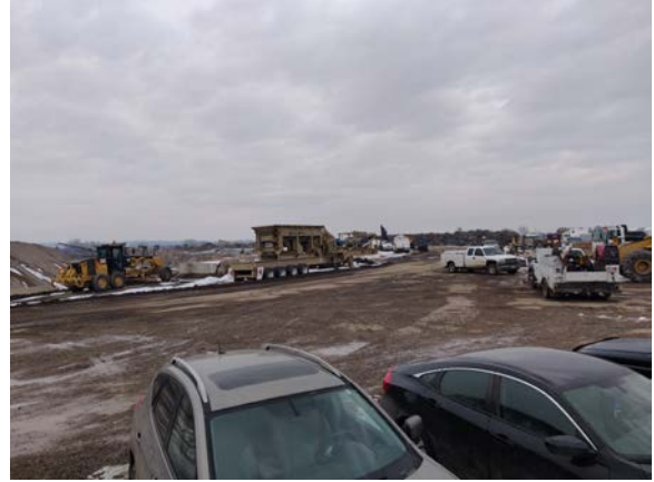
View of southeast area looking north shows road conditions are wet.
