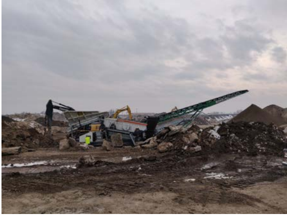
View of concrete crushing process (typical) looking south from the northern perimeter.
