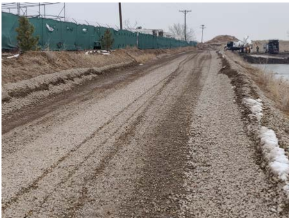
View of west perimeter road looking south. Melting snow reduced dusted generation from vehicles.
