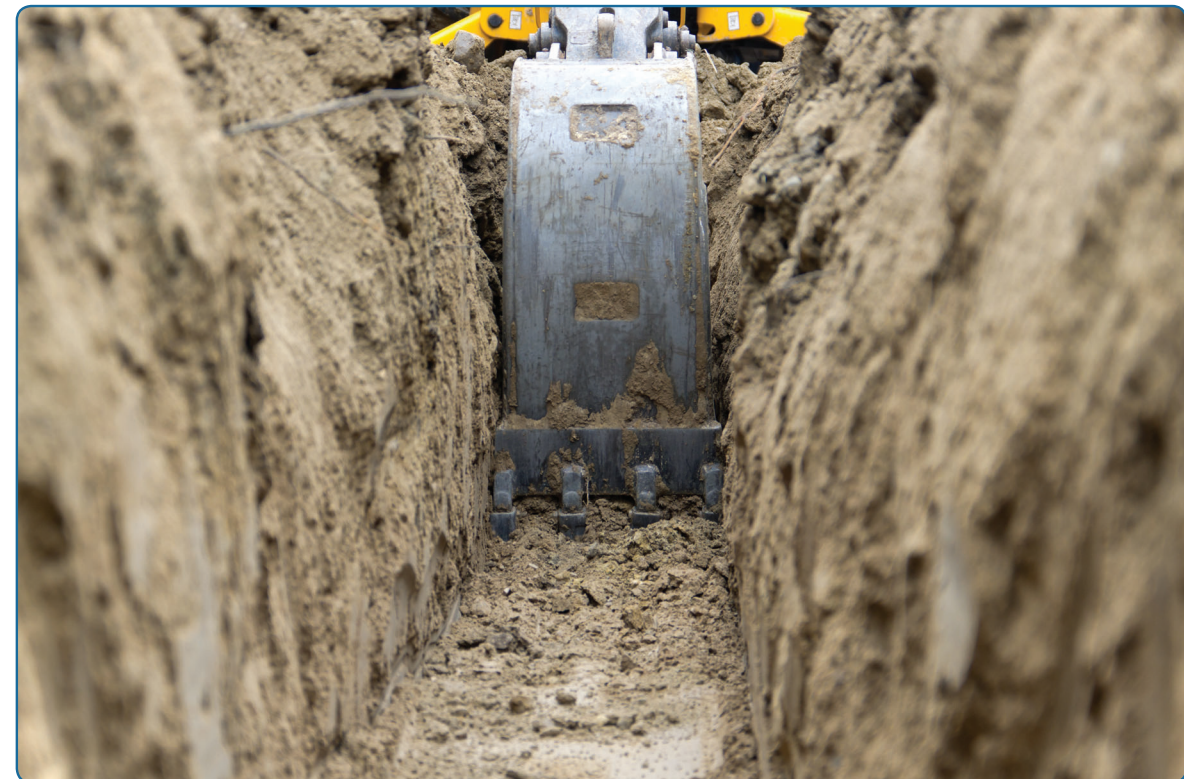
Pioneer is committed to safety at all stages of a project — from project initiation to pipeline operation and maintenance.
