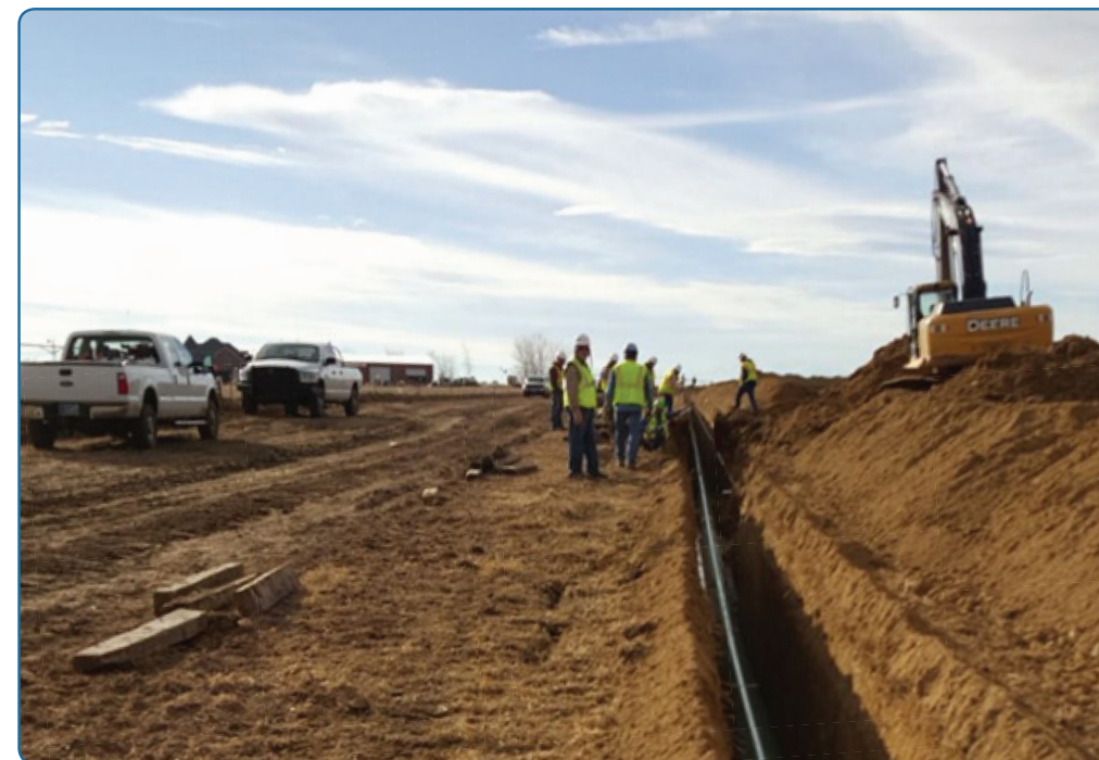
Pipeline joints being lowered into the trench. Post-construction, the right-of-way will be restored to the conditions required by permits and landowner agreements.
