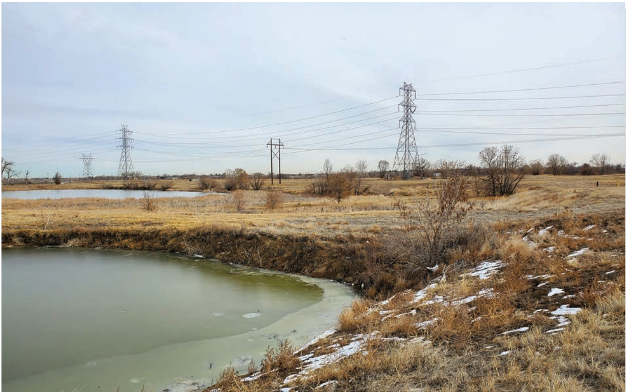
Photo 16 - Overview of AP2 Wetland 9 along AP2 OHWM 4. View is to the east.
