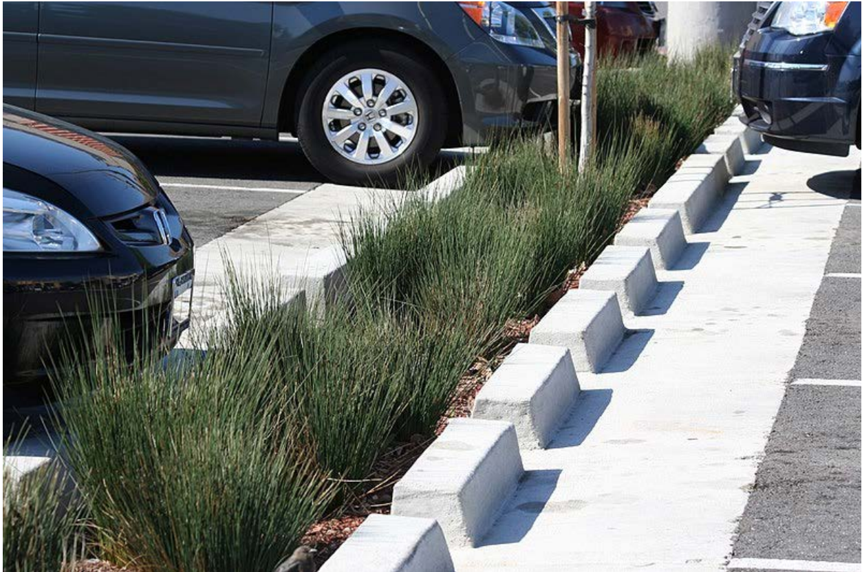
Bioswale w/ Non-continuous Curb
