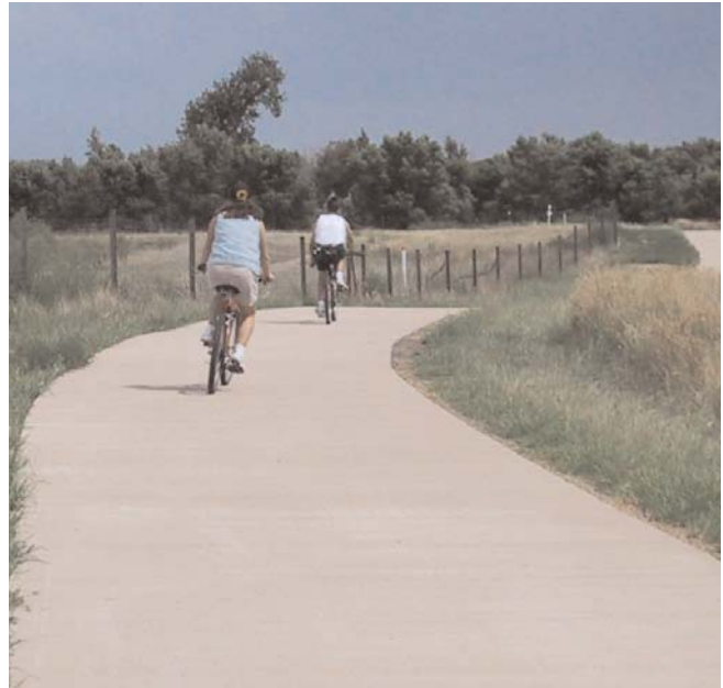
Existing Bike Path at 88th Avenue
