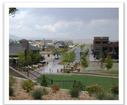
Mixed Use Neighborhoods include a range of urban-level residential and supporting uses.
